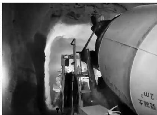
江西铜业 (武山三期) | KATG102 矿用混凝土搅拌机 UNDERGROUND CONCRETE-MIXER TRUCK WORKING UNDERGROUND IN THE WUSHAN PROJECT
