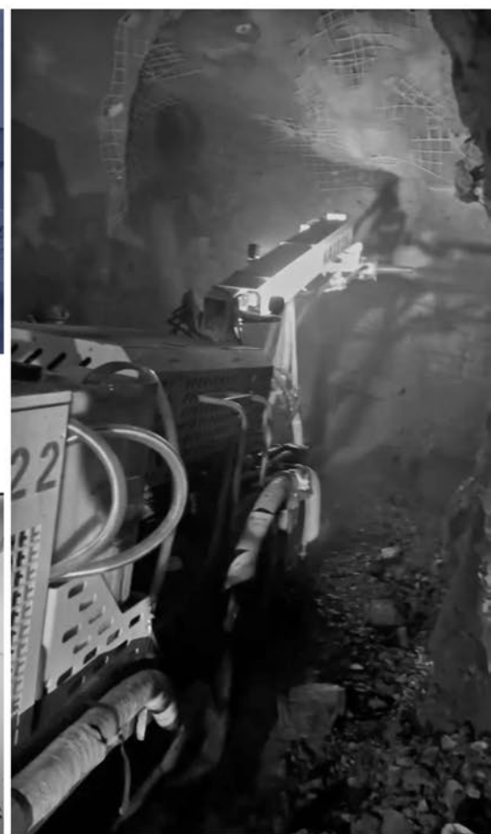
天一矿业 (瓮安项目) | KATP20 地下混凝土喷浆车 UNDERGROUND CONCRETE-GUNITING TRUCK WORKING UNDERGROUND IN THE WENGAN PROJECT
